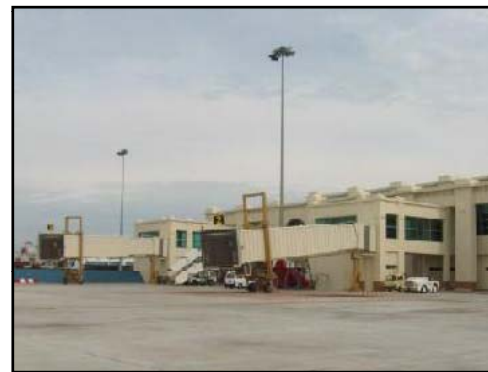
Aircraft Parking Apron and Taxiway
