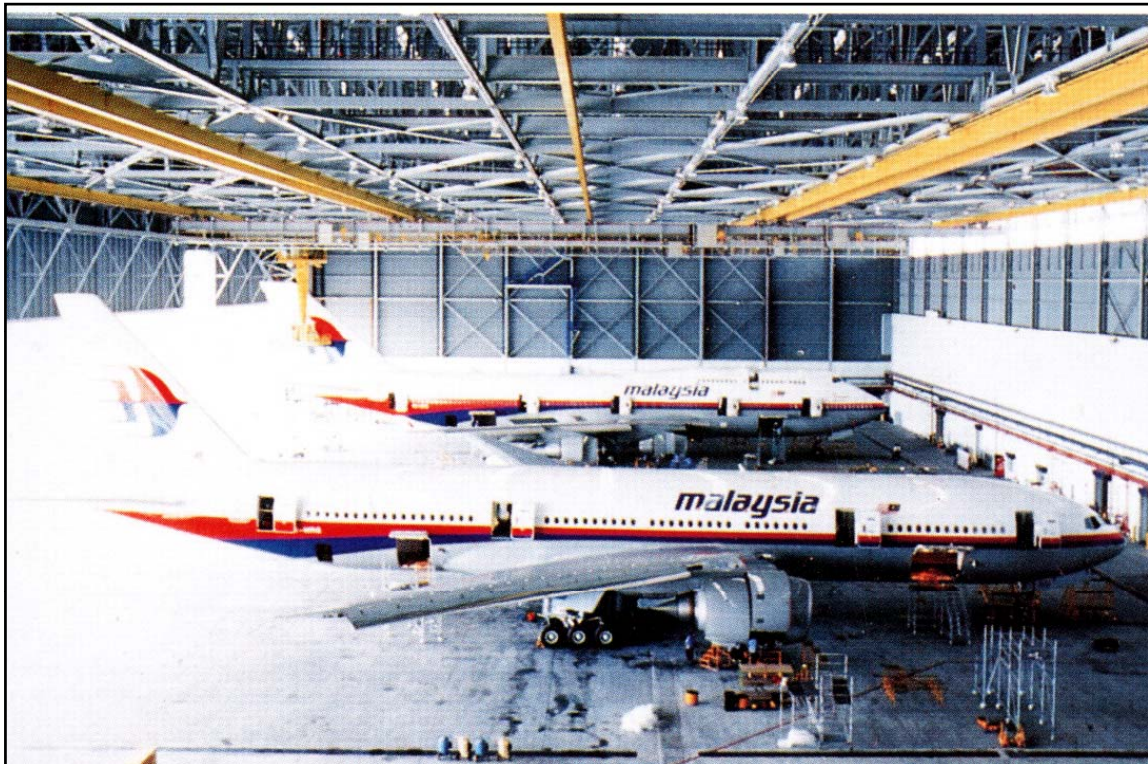
MAS Hangar & Hangar Shops
