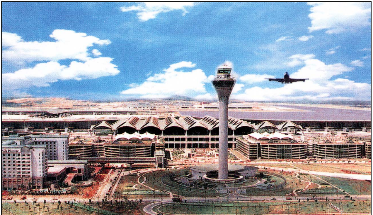
Airport Passenger Terminal Complex Contact Pier And Satellite Building
