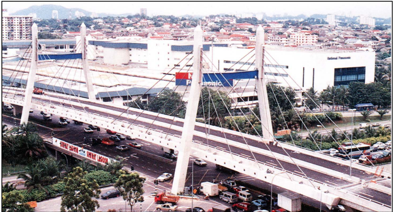
CABLE STAYED BRIDGE CROSSING THE FEDERAL HIGHWAY AT MOTOROLA
