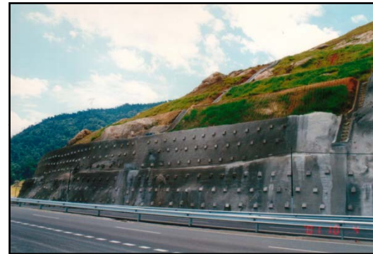
Construction of A Road in Very Hilly Terrain
