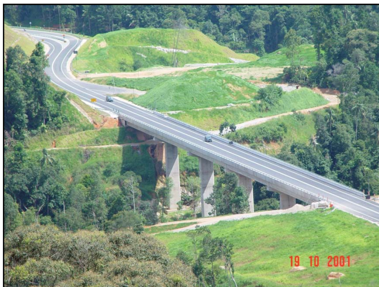
Overall View of 200 meter length Bridge over Sungai Selangor
