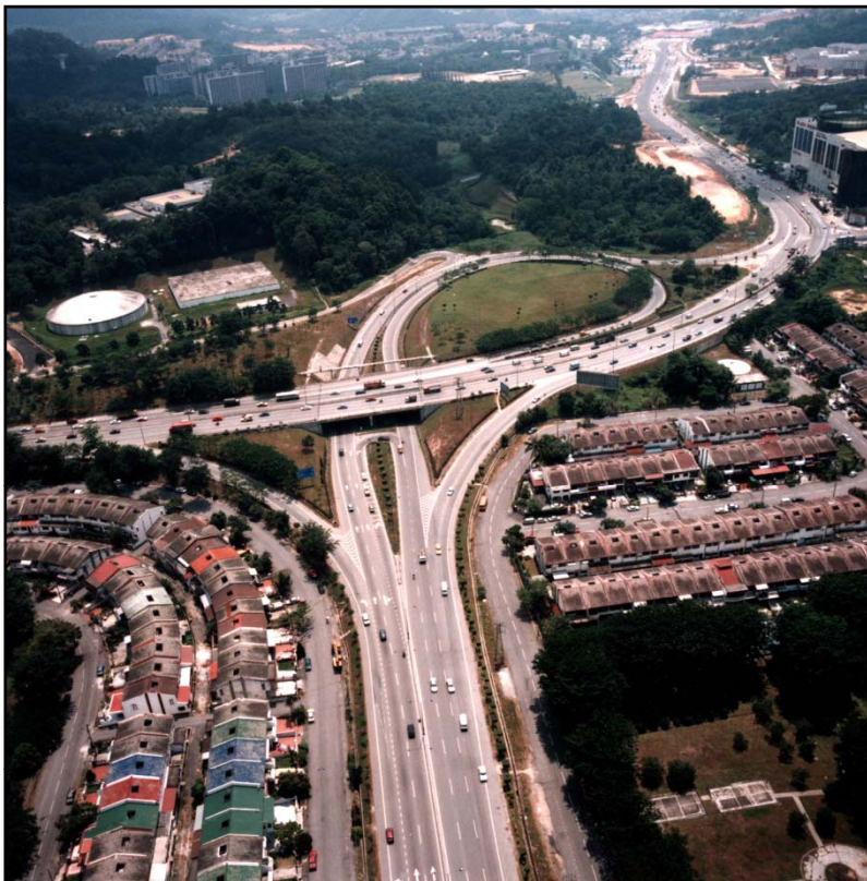
EAST-WEST LINK EXPRESSWAY
