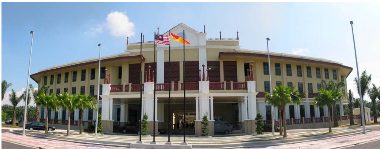
Kuala Langat Administrative Centre District Office
