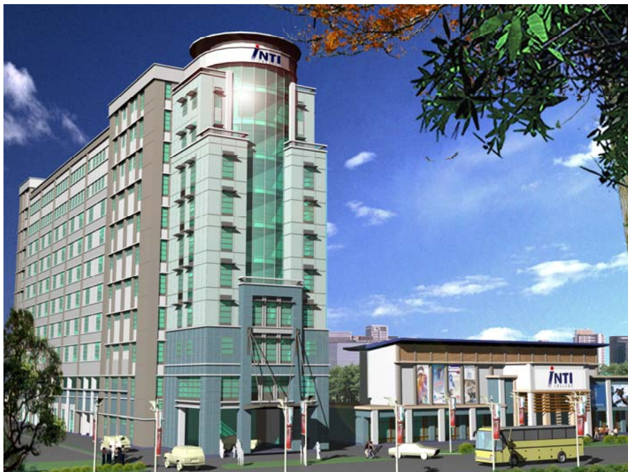
Re-Development of Inti College Subang Jaya (Phase 1)
