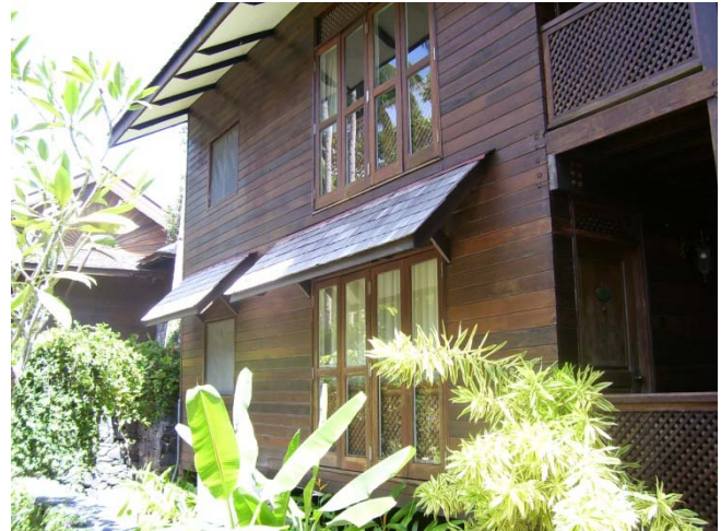
Existing Chalet House, Rebak Marina Resort
