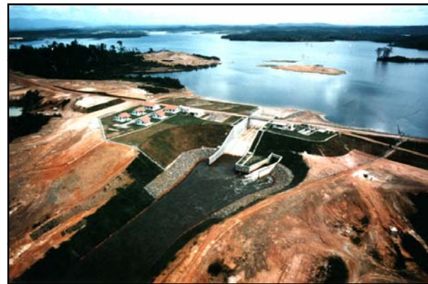
Earthfill dam 16m x 860m long with spillway
