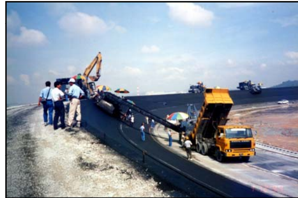
Work in Progress – Wearing Coarse (Final Layer)
