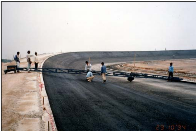
Dipping in Progress Checking Road Base Level
