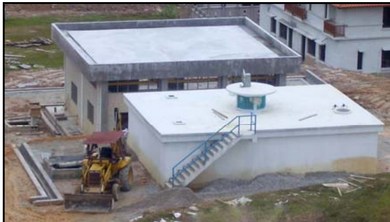
40,000 Gal. R.C. Suction Tank and Pump House
