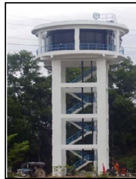
60,000 Gal. Elevated Permastore Tank and R.C. Water Tower
