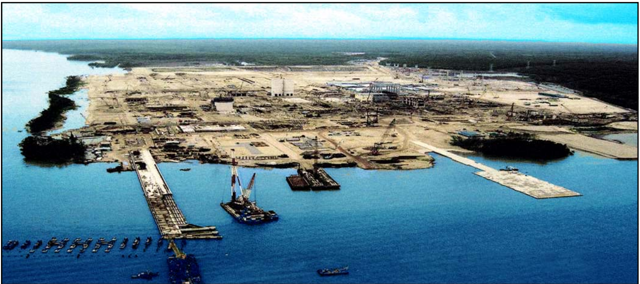
Plant during construction 2005
