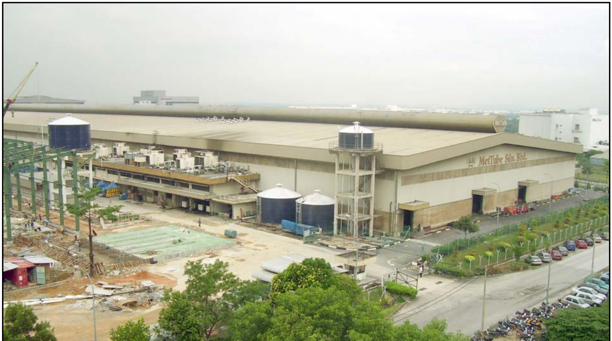
Copper Tube Factory, Shah Alam, Selangor
