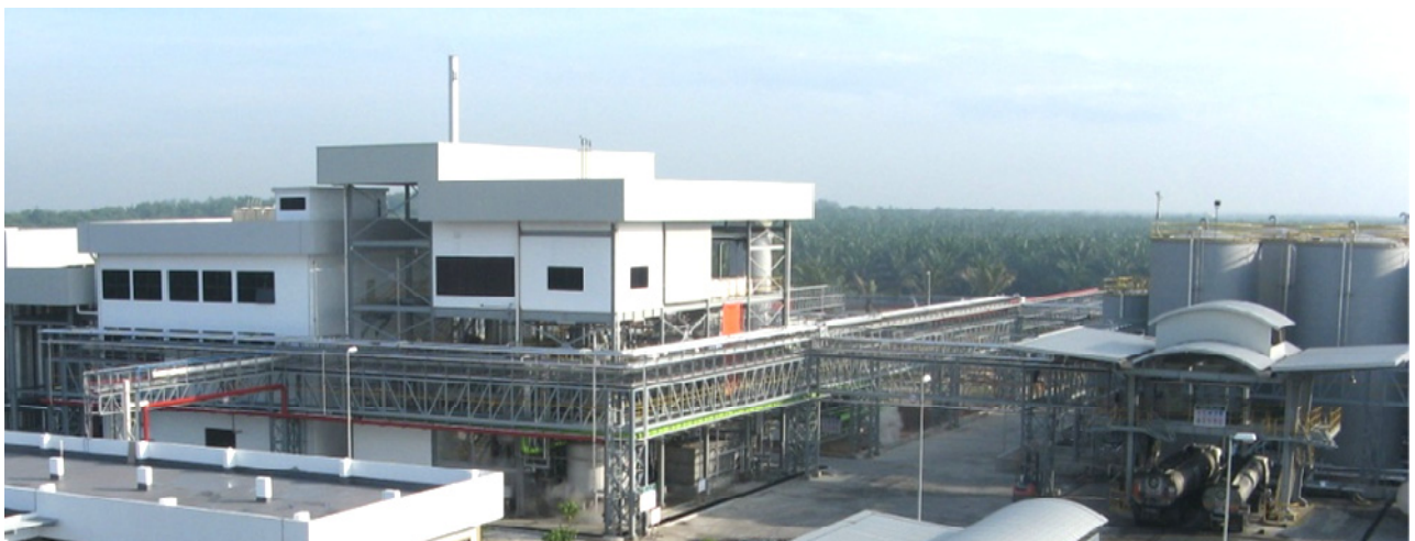
MPOB Biodiesel Plant
