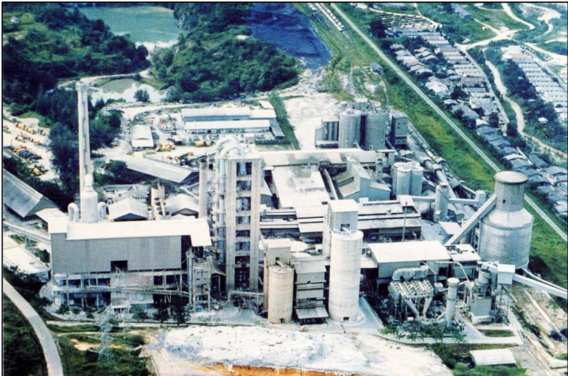
CEMENT PLANT RK3 3 RD KILN EXTENSION (4000 TPD), RAWANG
