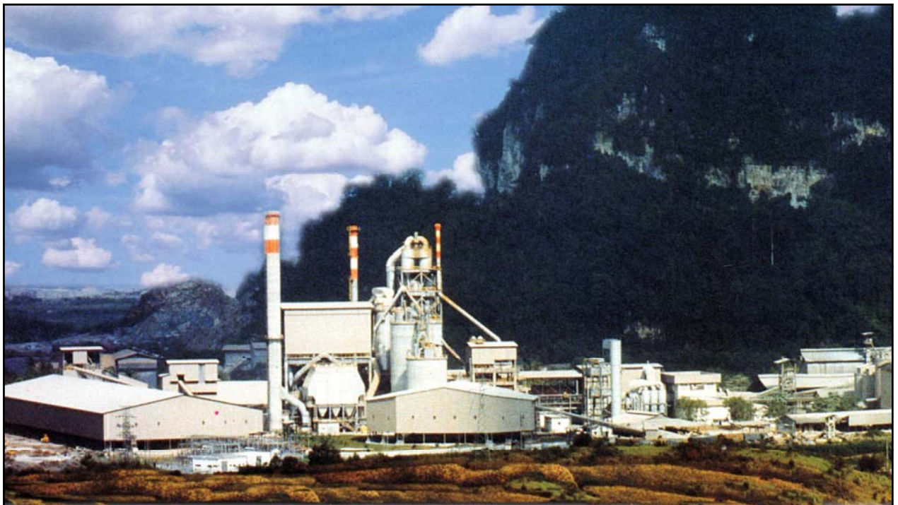
APMC, Kanthan KK3 (2000 TPD) Modernisation Works, Perak
