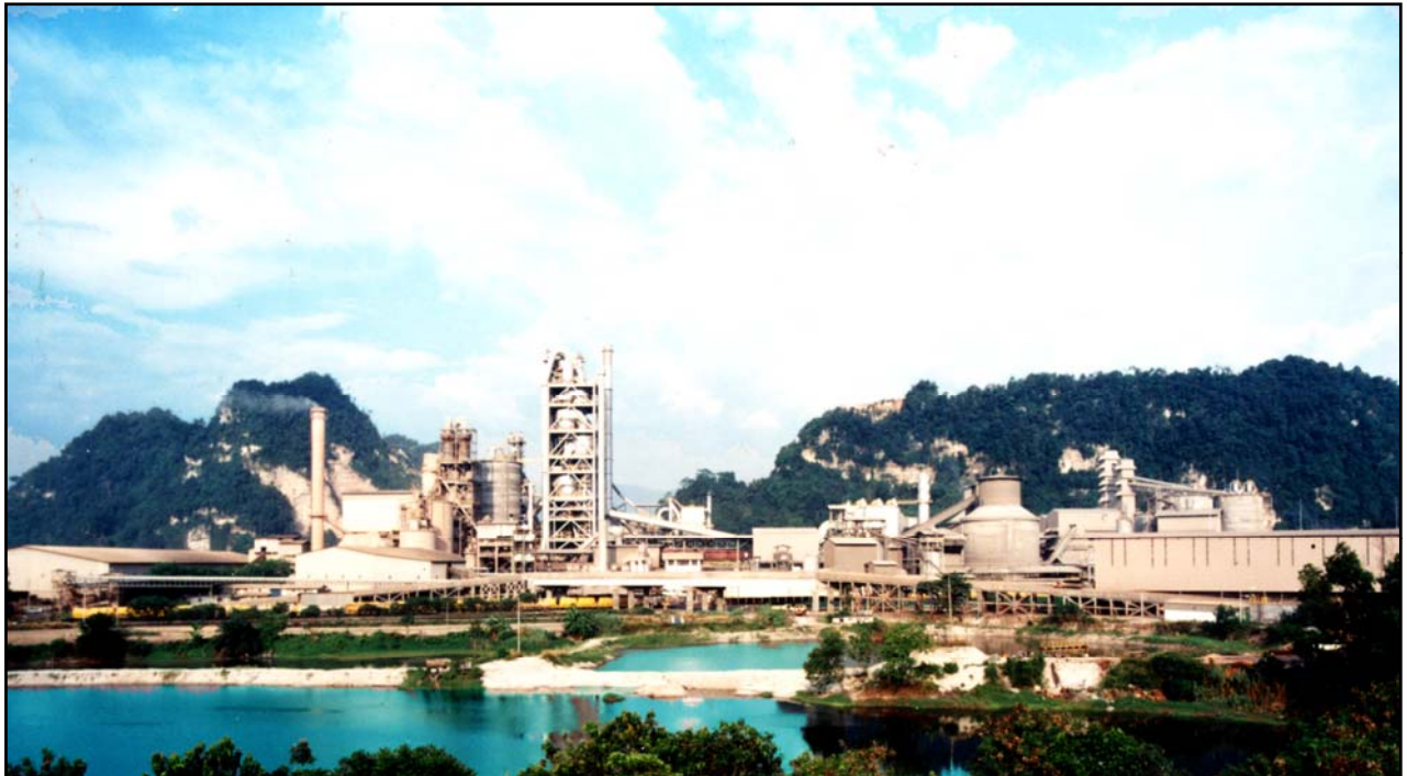
APMC, Kanthan KK4 (6000 TPD) Modernisation Works, Perak
