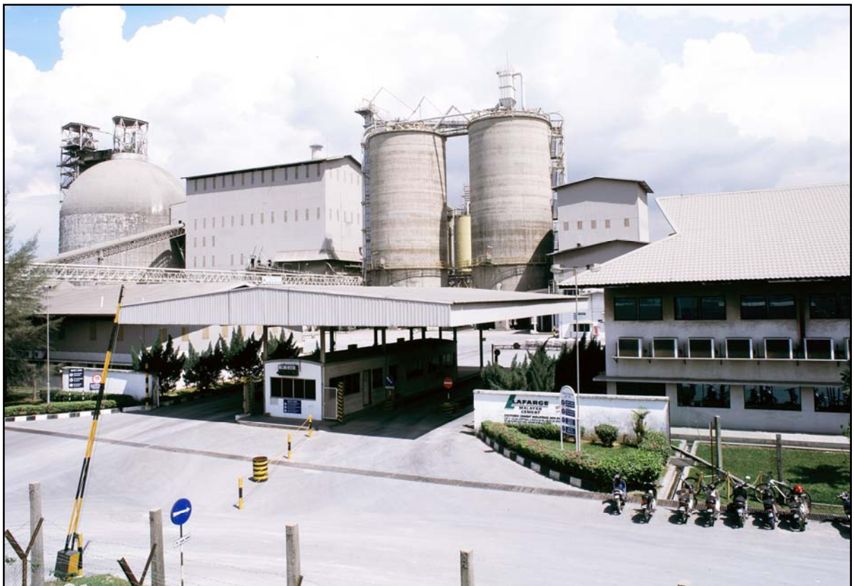
Cement Clinker Grinding Plant
