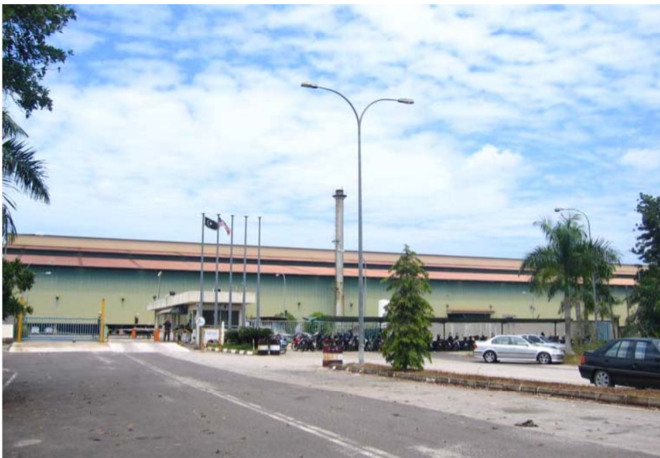
GIS Hot rolled Plate Mill
