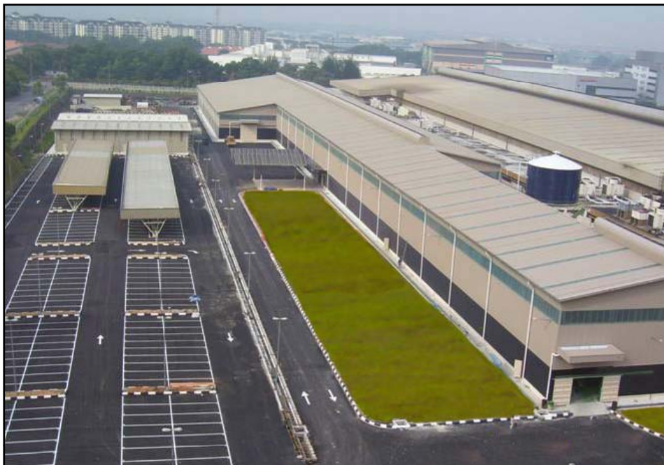
METTUBE FACTORY EXTENSION
