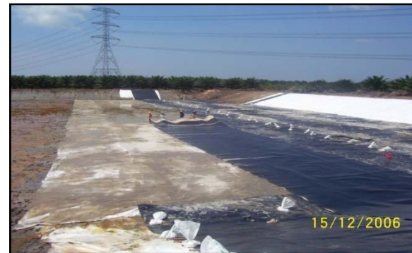
Geotextile Separator &amp; HDPE Liner for Landfill Cell
