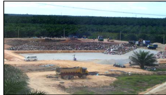
Overall View of Landfill
