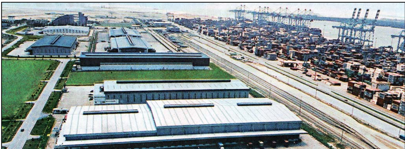
Rail Container Transfer Station at Pelabuhan Tanjung Pelepas, Johor
