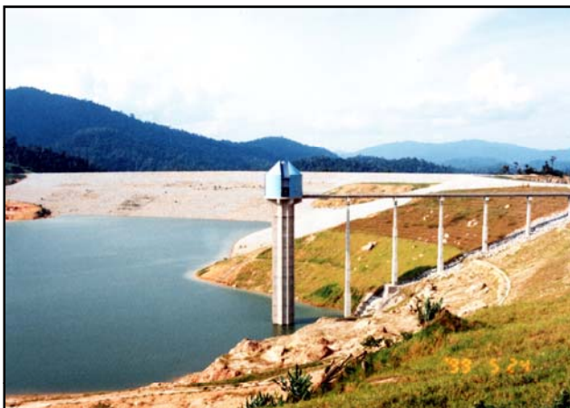
54m high by 554m long secondary dam in the foreground; 70m high by 270m long main dam at centre; and 72m high intake tower with access bridge on the right
