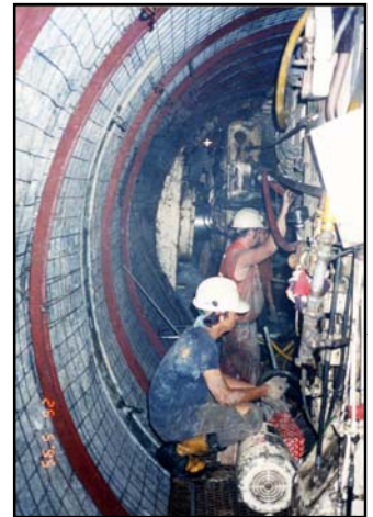
3.2m Dia. bored tunnel with tunnel boring machine
