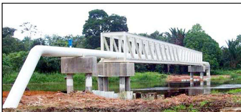
NEW 600MM DIA. MILD STEEL PIPE CROSSING SG. SIMPANG KIRI, BATU PAHAT, JOHOR
