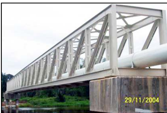
NEW 600MM DIA. MILD STEEL PIPE CROSSING SG. SIMPANG KIRI, BATU PAHAT, JOHOR
