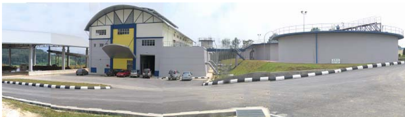
SLUDGE TREATMENT FACILITIES
