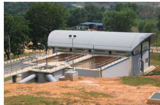
EFFLUENT HOLDING TANKS
