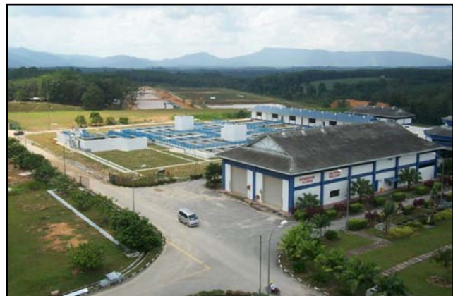
SG. JOHOR WATER TREATMENT PLANT
