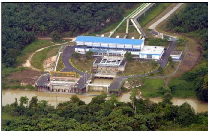
AERIAL VIEW OF SG. JOHOR INTAKE
