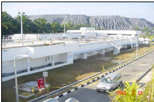
SEDIMENTATION &amp; FILTER TANK
