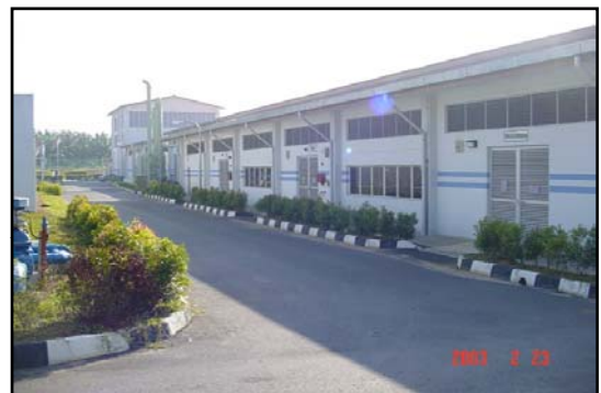
PUMP HOUSE &amp; CHEMICAL BUILDING
