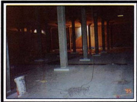
Interior of 32 MI Bukit Jelutong Balancing Reservoir
