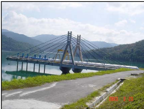
80m LONG CANTILEVERED CABLE STAYED FOR RAW WATER INTAKE
