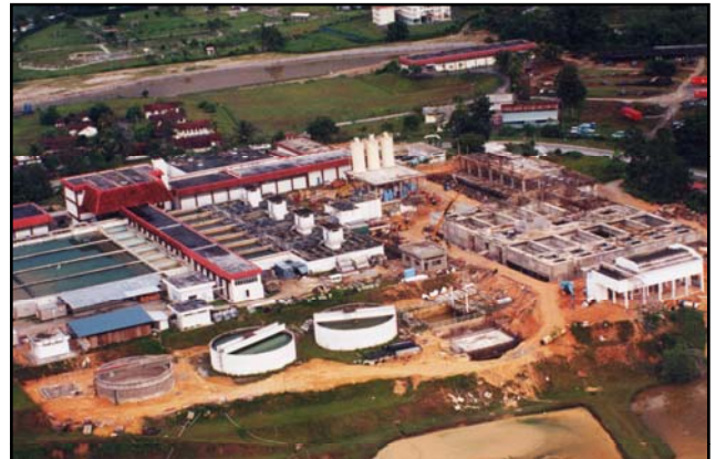
OVERALL VIEW OF SG. TERIP WTP
