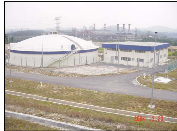
4.5ML R.C. SUCTION TANK AND PUMPHOUSE IN PRECINCT 11
