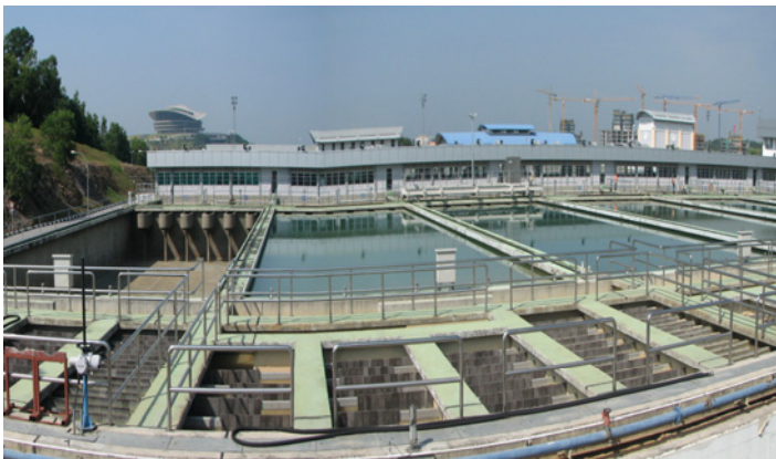
View of Filter and Sedimentation Tanks
