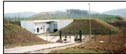
Typical Completed Sunken Pump Station
