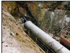
Laying of 900mm dia. D.I. pipe in progress
