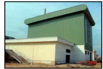
View of Sludge Dryer
