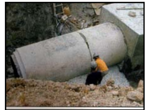
Filling of Granular Material to 1500mm dia. pipe trench
