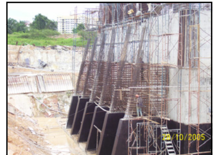
CONSTRUCTION PUMP STATION EXTERNAL WALL IN PROGRESS
