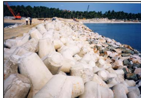
Northern Breakwater Under Construction
