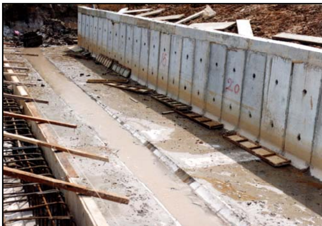
Outlet channel from road culverts
