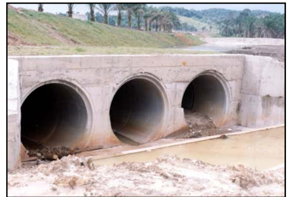
Road culverts crossing Road D
