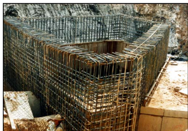
Manhole construction at main drain
