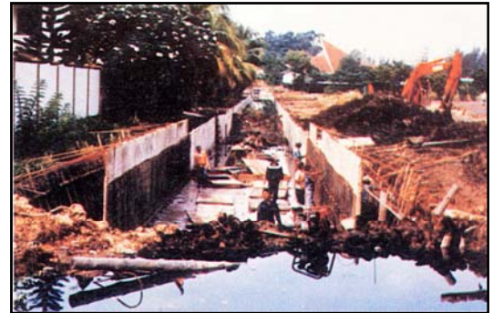
RC Drain under Construction
