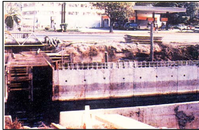
Triple Cell Culvert at Drain Junction
