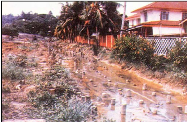
Piling Works along Drain Alignment
