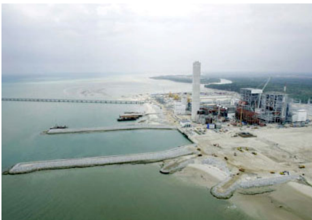
Overall View of the Plant
