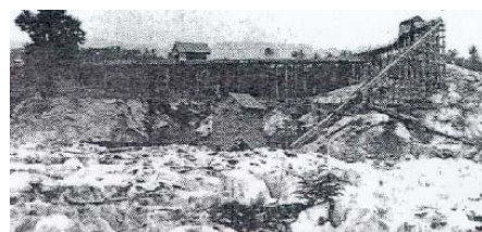
Fig. 3 Palong in an opencast tin mine in Segambut (Gobbett, 1973)
