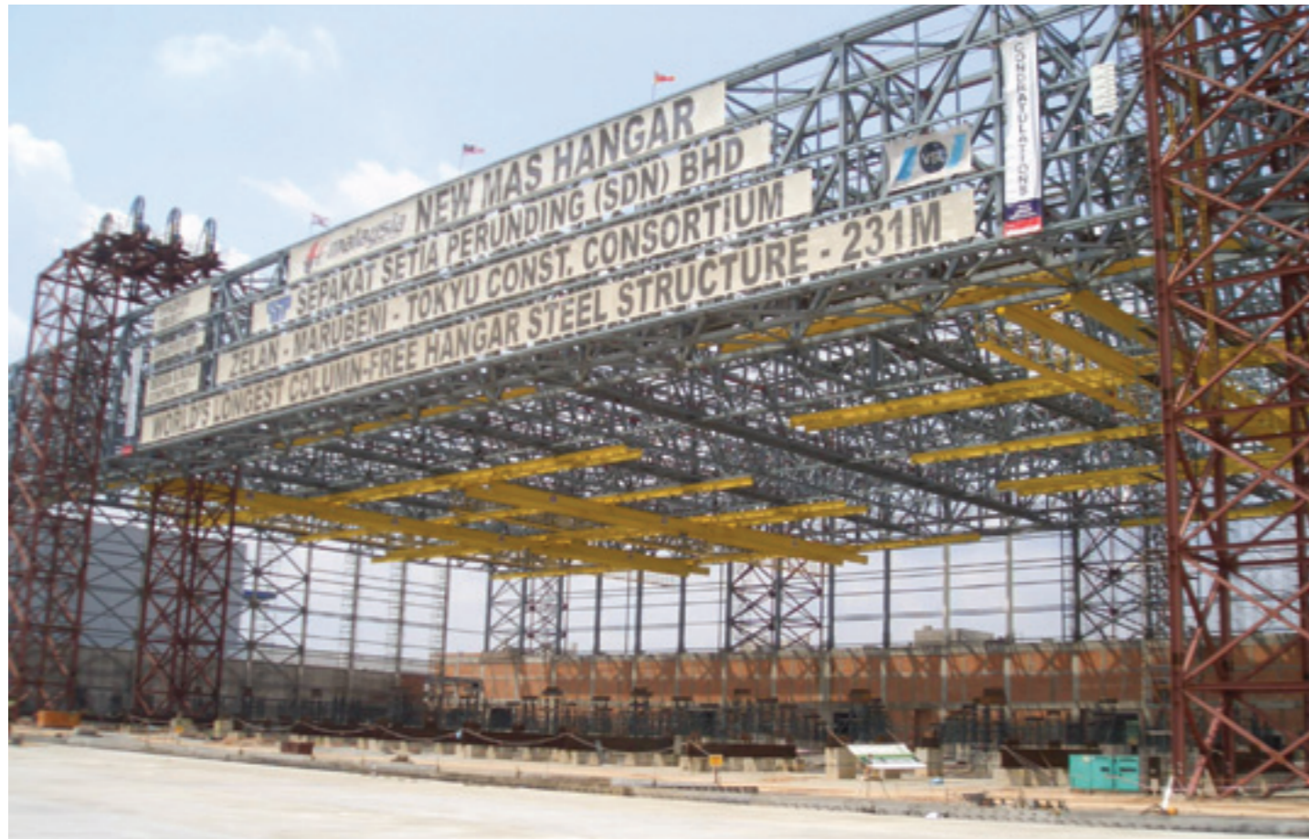
Figure 11: Hangar roof structure lifting in progress
