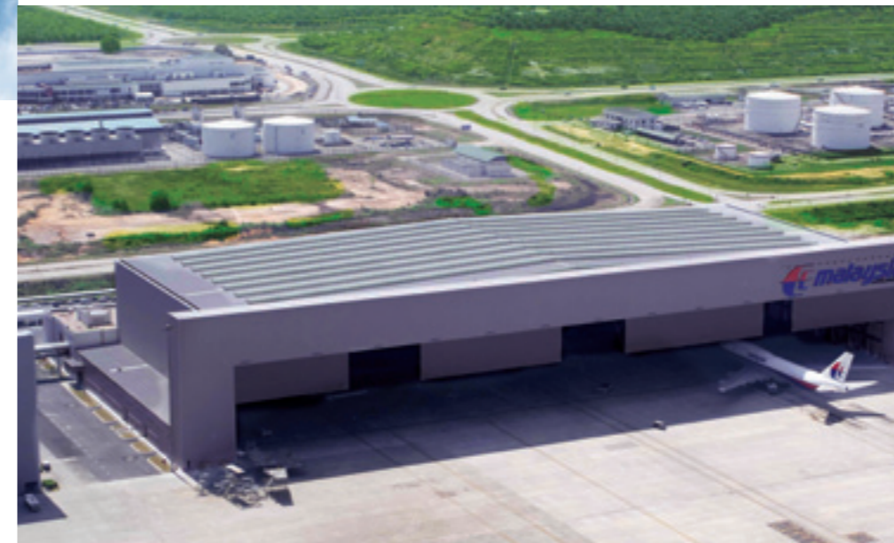
Figure 2: Photograph of the completed hangar
