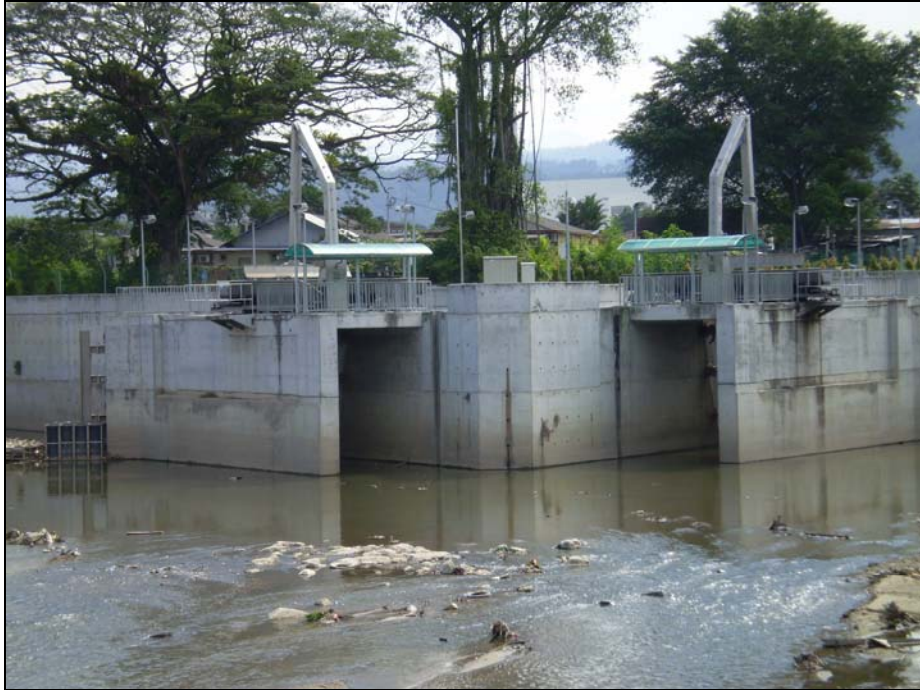
Figure 3: The Debris Removal Systems for Sg Ampang & Sg Klang Situated at the Confluence of the Two Rivers
